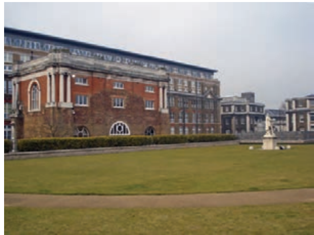
Green roof at Woolwich Royal Arsenal
